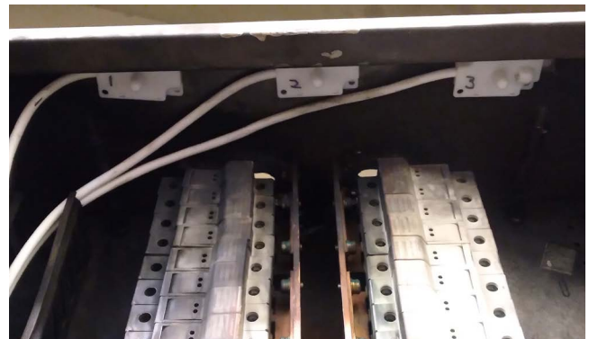
FIGURE 7. Approximate location of the light sensors inside the panel (left) and the light sensors at the top of the enclosure (right).
